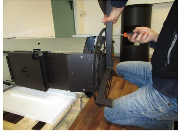
**Fig. 48 - Secure the bench pedestal**
