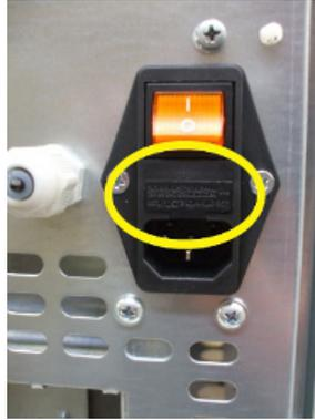
*Fig. 106 - Shutter with fuses to remove*
