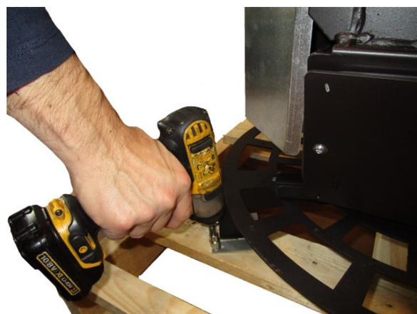
**Fig. 34 - Bracket removal**
